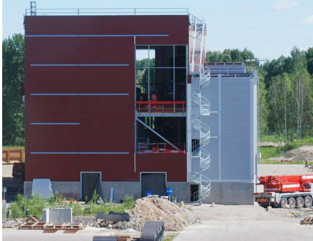
The building is starting to take shape.
