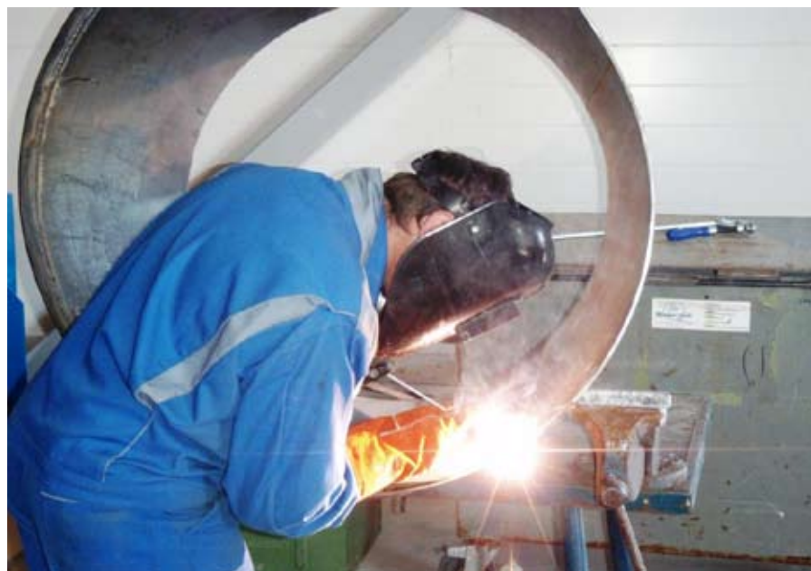
German company Kramer & Best is doing the welding.
