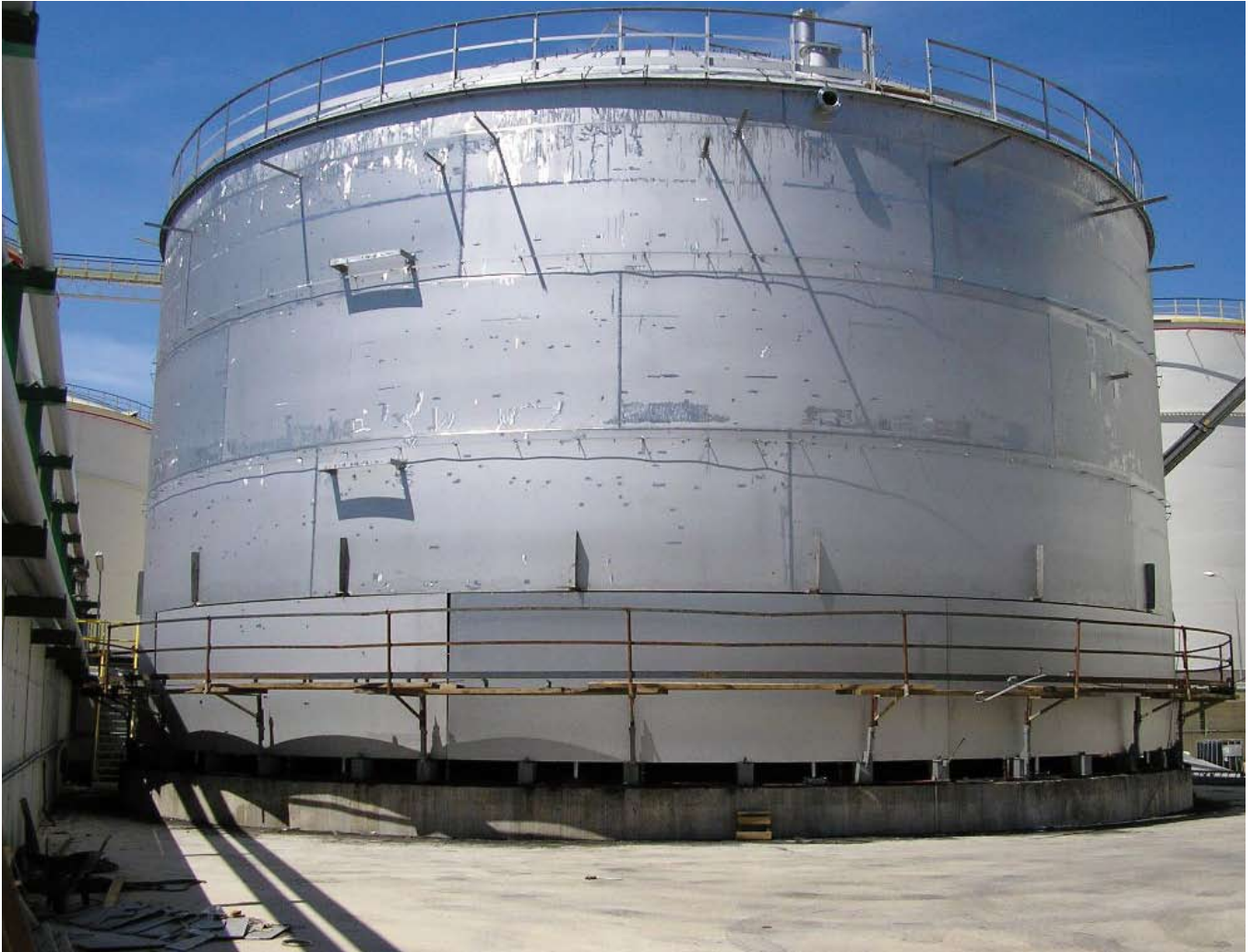
Figure 4: A pickled, duplex 2304 storage tank
