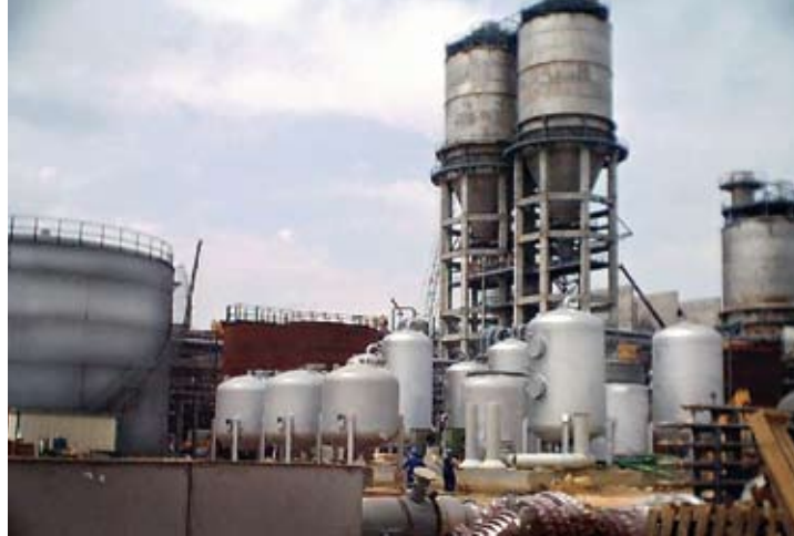
Figure 2: Treated and untreated stainless steel tanks
