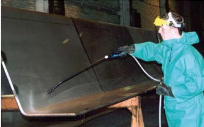
Figure 17: Passivation of what will be part of a chemical tanker bulkhead in duplex stainless steel
