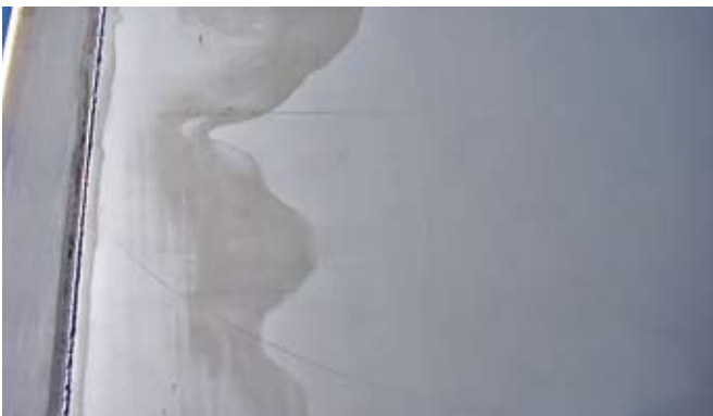
Figure 21: Water staining
